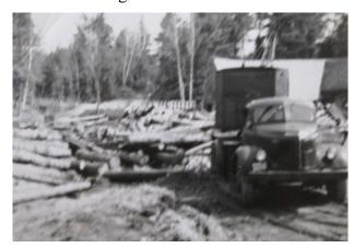
This 1950's truck had a crane on its flatbed and was used to clear the logs to be able to rebuild the road.
