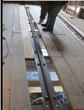
Left: The track is absolutely straight and level. Scott is cutting boards to fit in the spaces between the track and the floor.
