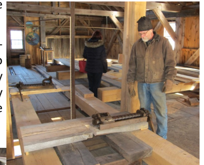
Left: The track is absolutely straight and level. Scott is cutting boards to fit in the spaces between the track and the floor.
