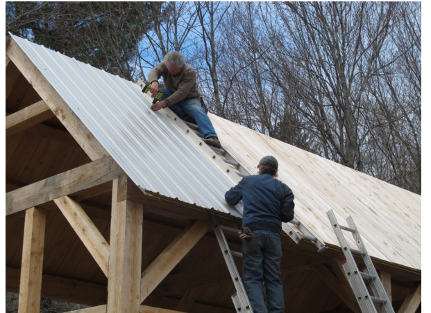
Top left: Crew who helped stand the shed. Top right: Putting the roof sheathing on. On the right: Installing the metal roof. On the left: Good days work with the siding in place and door on.
